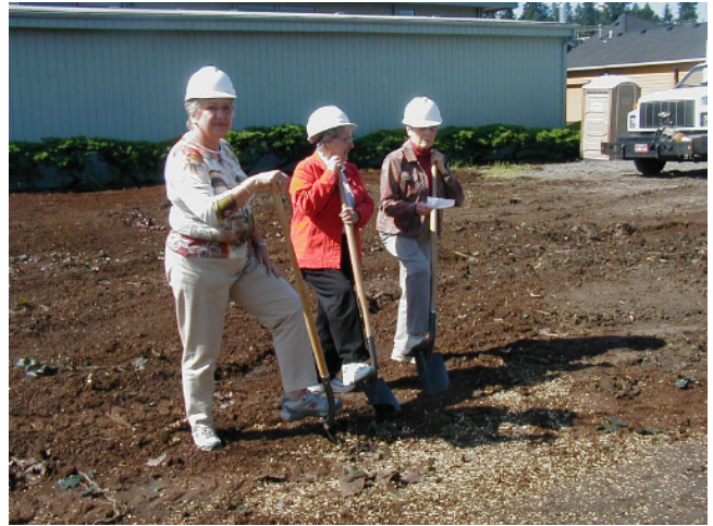
The Ground Breaking
