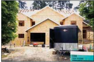
Duplex 1 is being sheeted and roofed.
