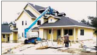
The four-plex will be completed soon.
